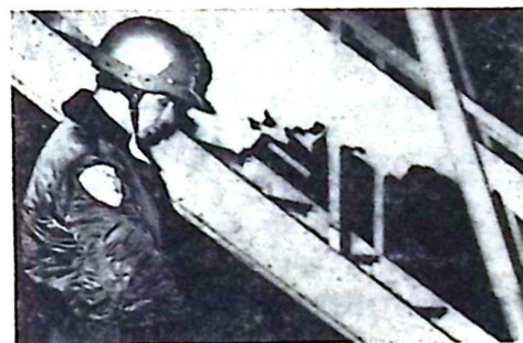
Checking the exit ramp at Reno
